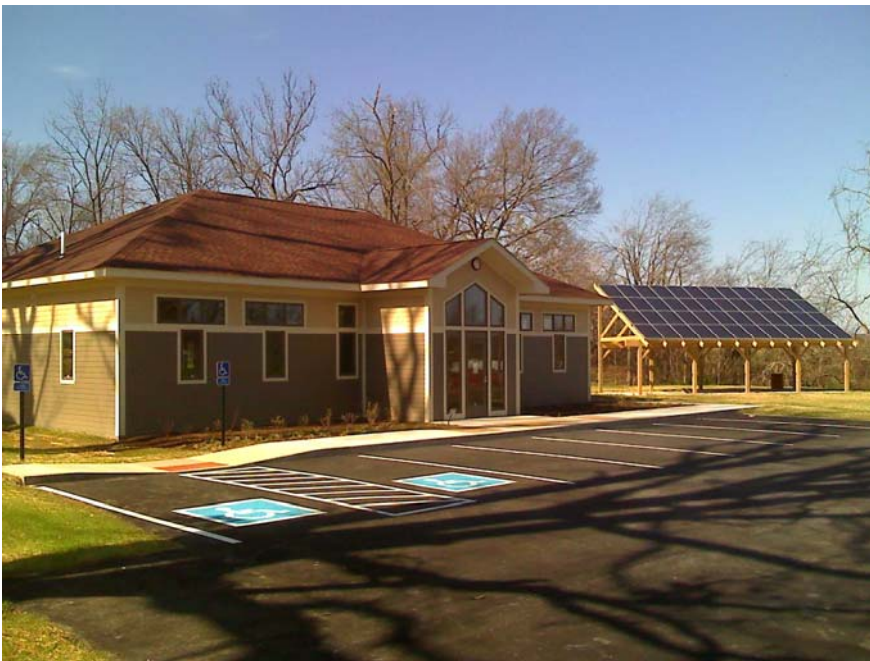
9KW Grid-Tied Solar System installed at Chrisney Public Library in Chrisney, Indiana. First Net-Zero energy library in Mid-West. Owner: Town of Chrisney 22 E. Chestnut St, Chrisney, IN (812)362-8668 Completed Dec. 2008
