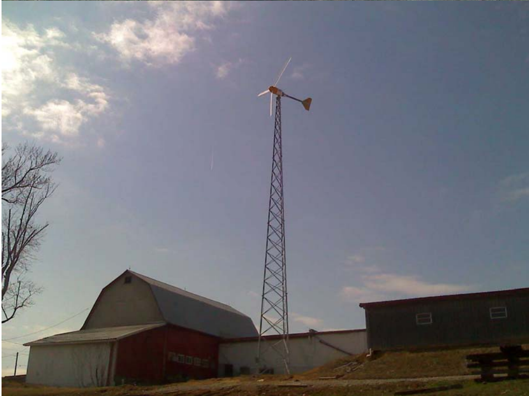
Bergey Excel-S 10KW Wind Turbine on 80' tower located at Engelbrecht Orchard in Evansville, Indiana. Completed: Feb. 2009. Owner: Connie Engelbrecht (812)423-1079
