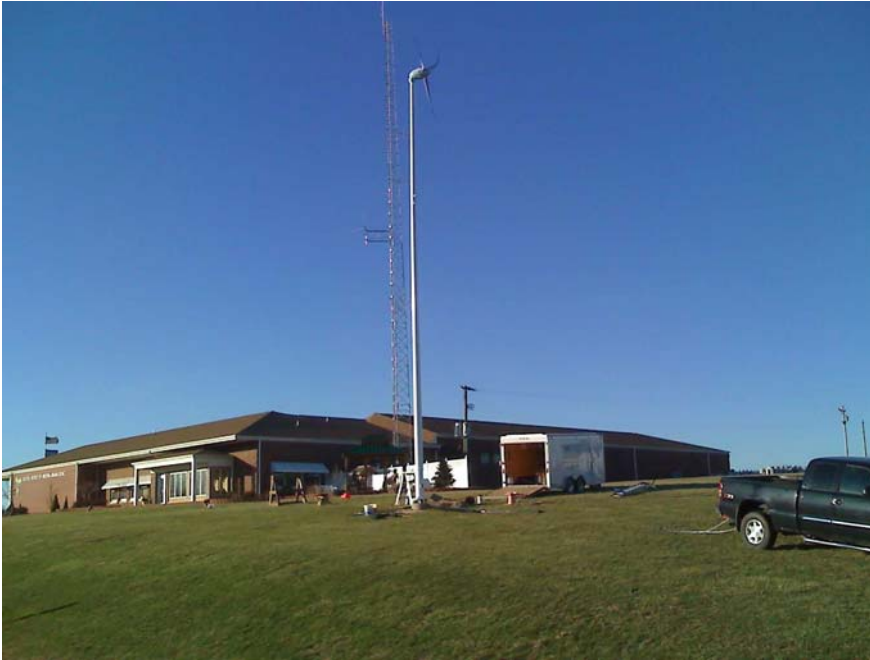
Skystream 3.7 on 50' Tilt-up Tower installed at Utilities District of Western Indiana (UDWI) REMC in Bloomfield, Indiana (812)384-4446
